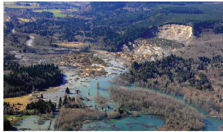
SR 530 Emergency Reconstruction DB (Oso Landslide), Environmental Permitting, Wetland Mitigation and Design, Oso, Washington, U.S.
